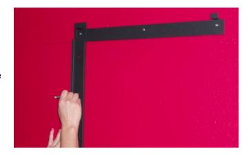
Remove the bracket and drill the newly marked holes. Tap into each hole one plastic wall anchor.
